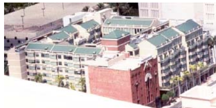
A rooftop view of Honuakaha.
